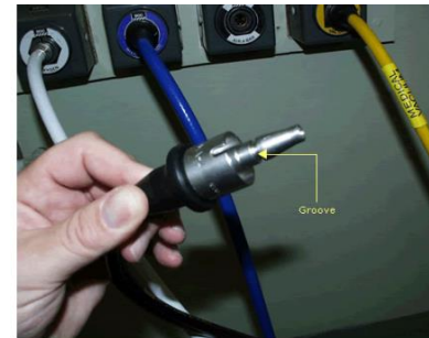
Fig 2 Groove in probe
