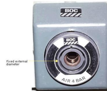
Fig 6 MA4 outlet showing fixed external diameter
