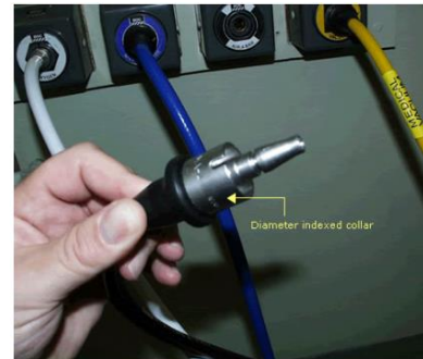
Fig 3 Diameter indexed collar
