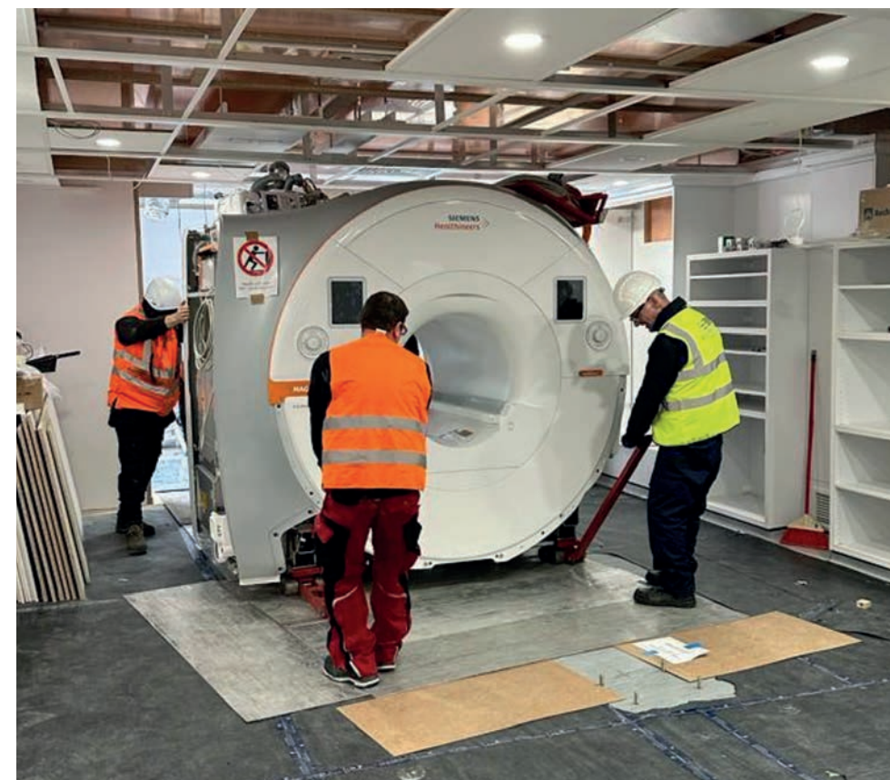
Installation of the new MRI scanner.
